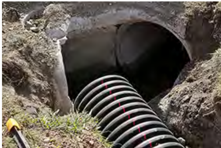
UPGRADE OF STORMWATER DRAIN EDWARD STREET
