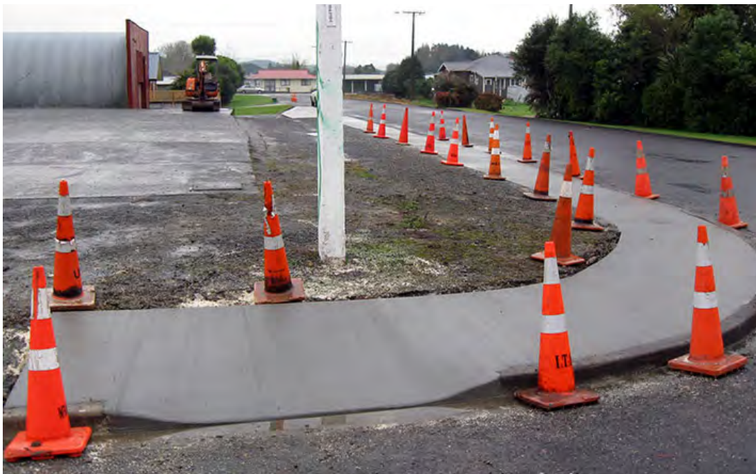
FOOTPATH RENEWAL WORK COMPLETED ON HIKAKA AND WARD STREETS, TE KUITI
