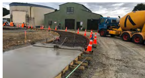
NEW DRIVEWAY TO SITE
