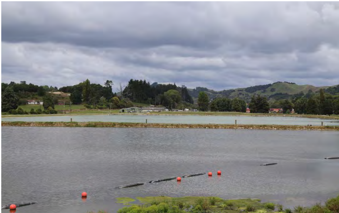
PONDS AT TE KUITI WASTEWATER TREATMENT PLANT
